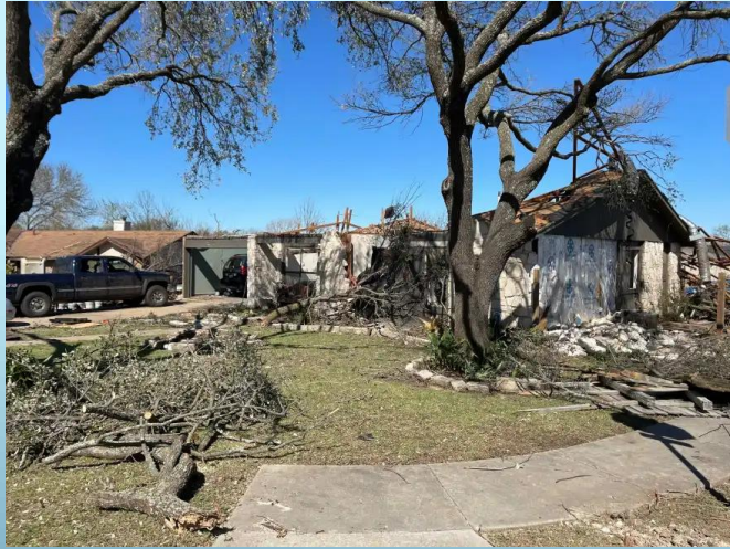
The front of Talamantez' home in Round Rock after a tornado came through on March 21, 2022. (KXAN Photo/Maggie Glynn)
